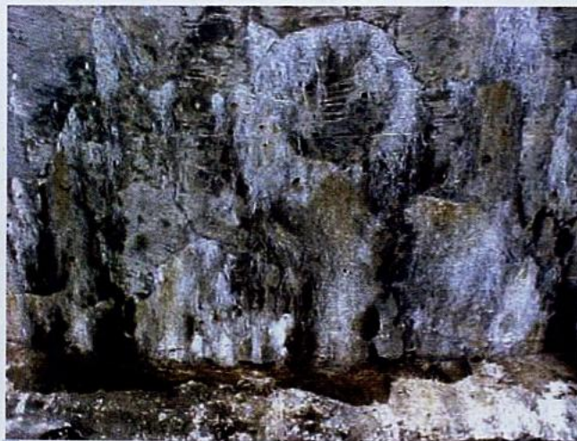
Original ferrocement reservoirs showing extensive leaks, cracks and sprawling of reinforcing internally
