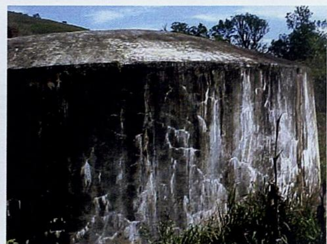
Original ferrocement reservoirs showing extensive leaks, cracks and sprawling of reinforcing internally
