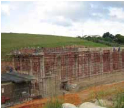
Figure 1: Overall view of the Booster Pump Station
