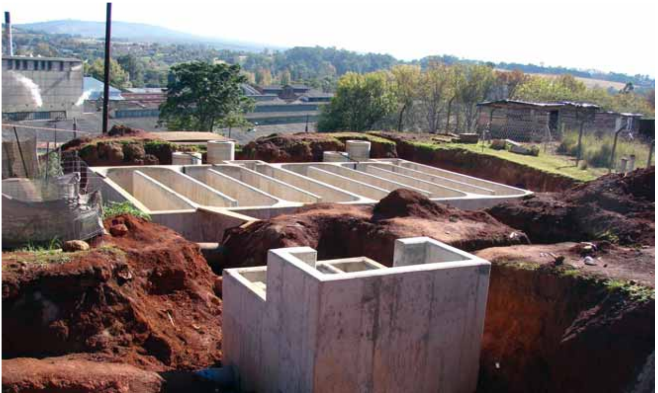
The new chlorine contact tanks and splitter chamber nearing completion. Excavation around splitter chamber and in coming pipework was undertaken by hand. The existing chlorine tank surround with Hessian cloth can be seen on the left of the photo.
