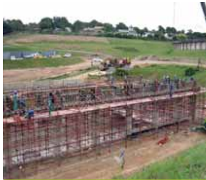
Figure 2: View of ring beam at northern end of pump station
