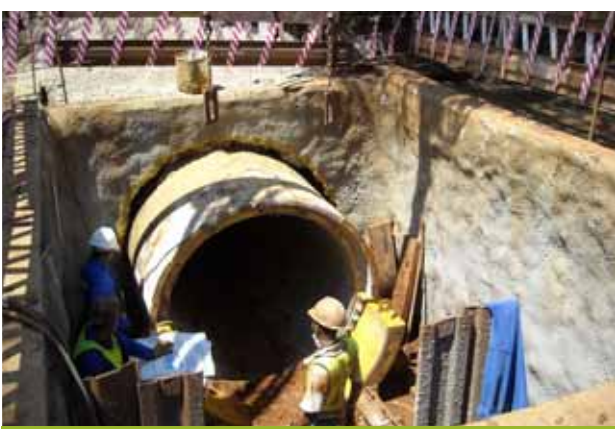
Jacking under R103
