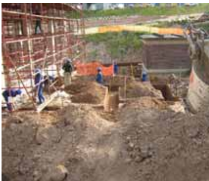
Figure 4: Strip footing foundation excavated for Transformer and of Switch room
