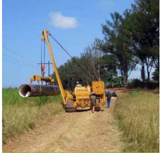
Moving Pipe using Side-Boom
