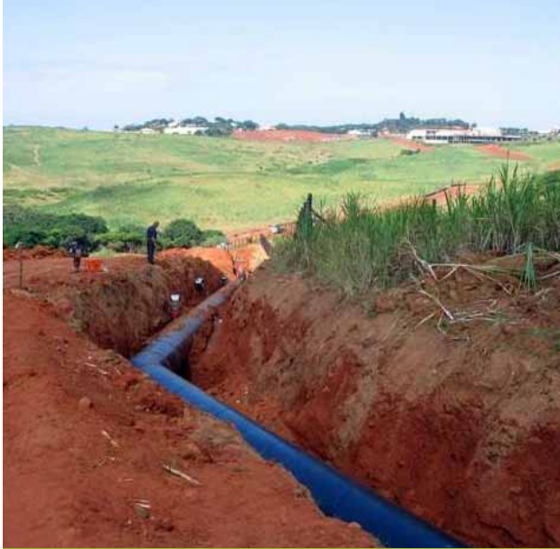
Pipeline looking down from Wakenshaw
