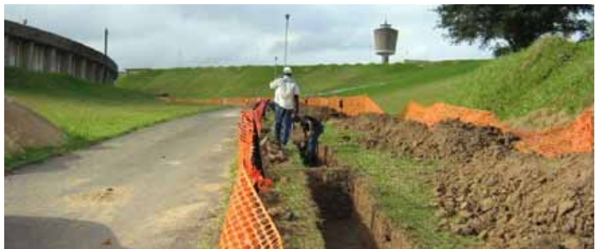
Figure 5: Trench excavated for street lighting and fibre optic cable installation
