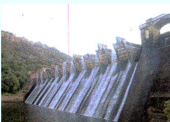
Completed in 1927, the Shongweni Dam holds back water from three rivers and served as Durban's main water supply for several decades. It was shut down in 1992 after the water capacity was reduced by huge volumes of soil and silt during a series of floods.
