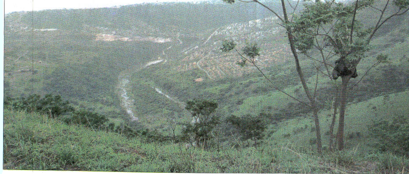
ROUTE: Down in the valley is the point at which the project team for the Western Aqueduct project has encountered the most challenges. The pipes will run down the slope on the right, through the river, and up the cliff on the left.
