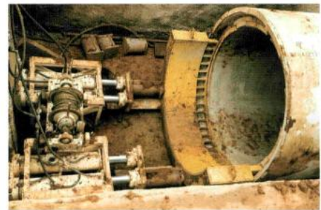
RIGHT View of jacking pit showing jacks, jacking ring and concrete sleeve
