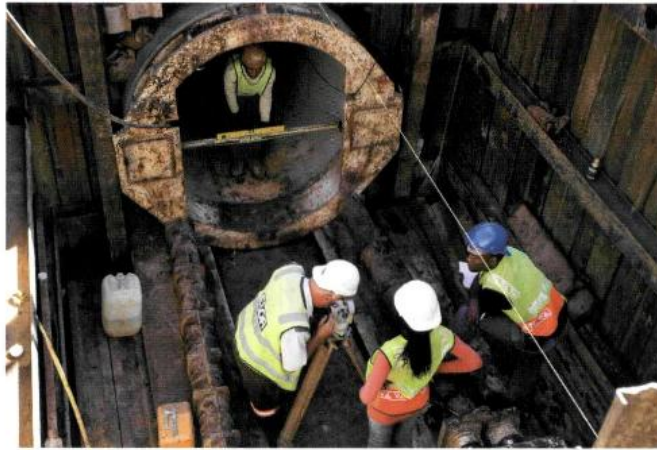
ABOVE Line and level control of pipe-jacking operation
