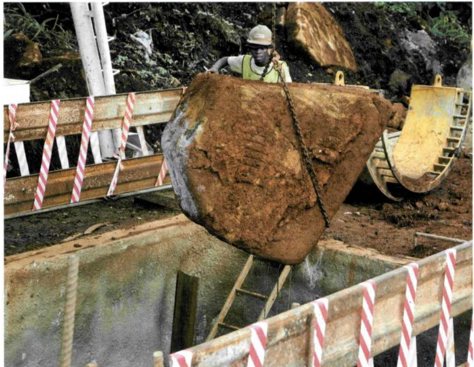
ABOVE Boulders removed from inside jacking sleeve
