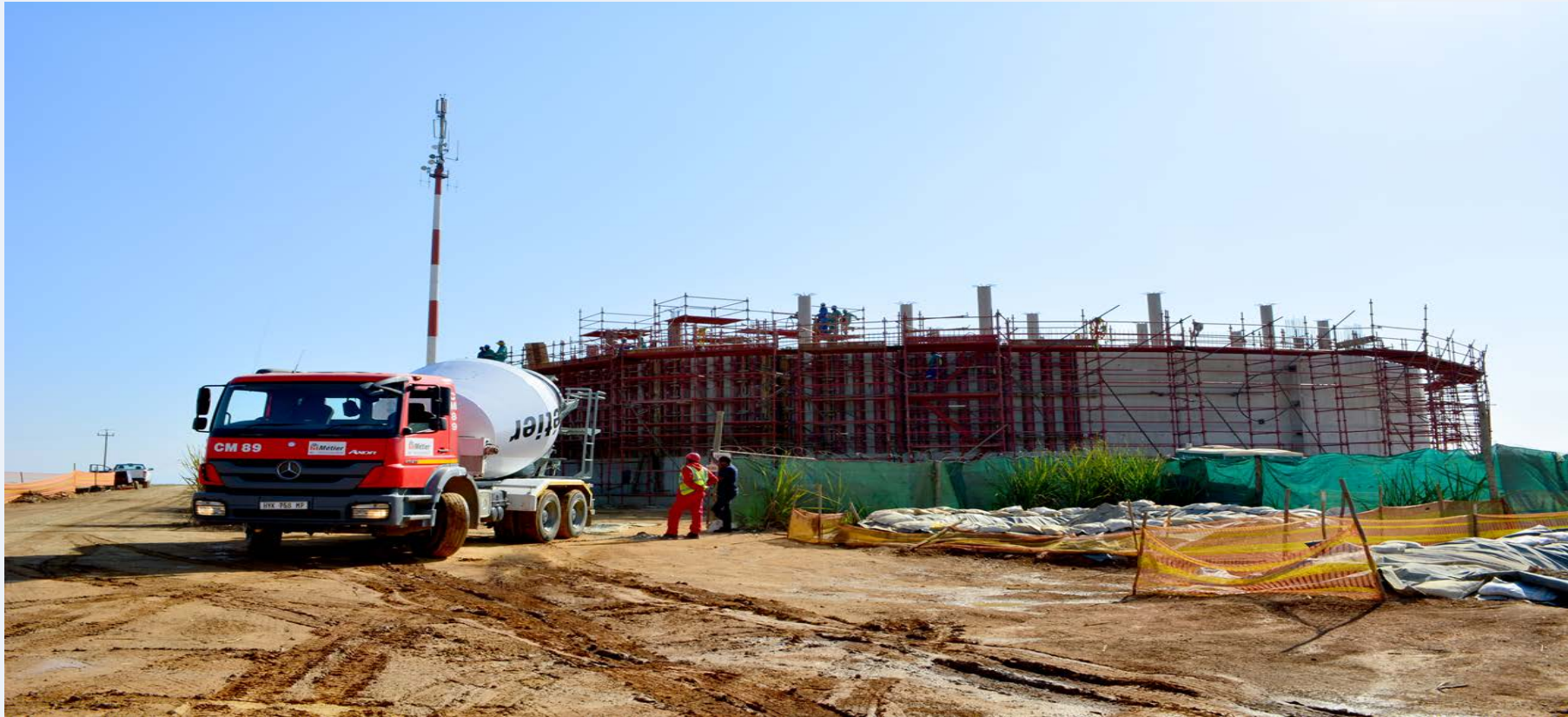
Mshwathi Bulk Water Supply project
