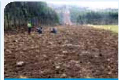
**(c)** Top soil removed prior to excavating the pipeline trench- note large sods which will be reset once pipeline is completed.
