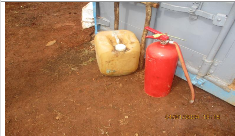
Figure 3: No drip tray under the petrol container
